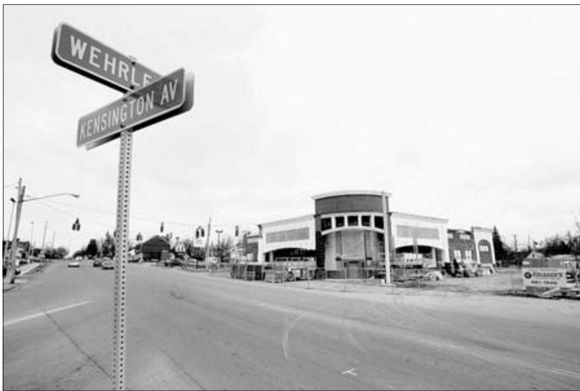
The intersection at Wehrle Drive and Kensington Avenue will be reconstruction into a roundabout, one of two being built at Harlem Road where the towns of
